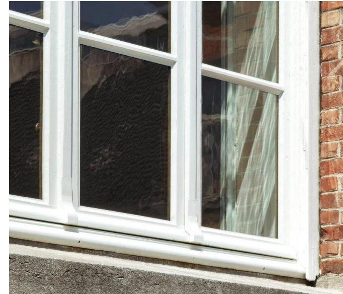
Vacuum glass FINEO – 0.7w/m 2 k
